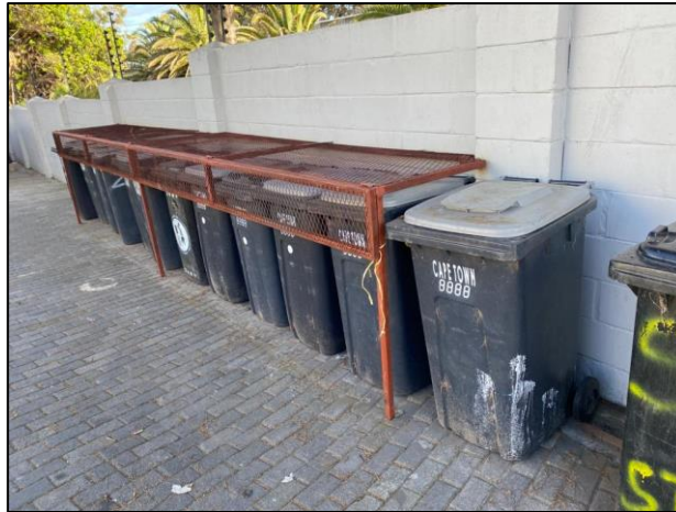
Figure 5. Bin housing area at Unit 10 Heron Park
